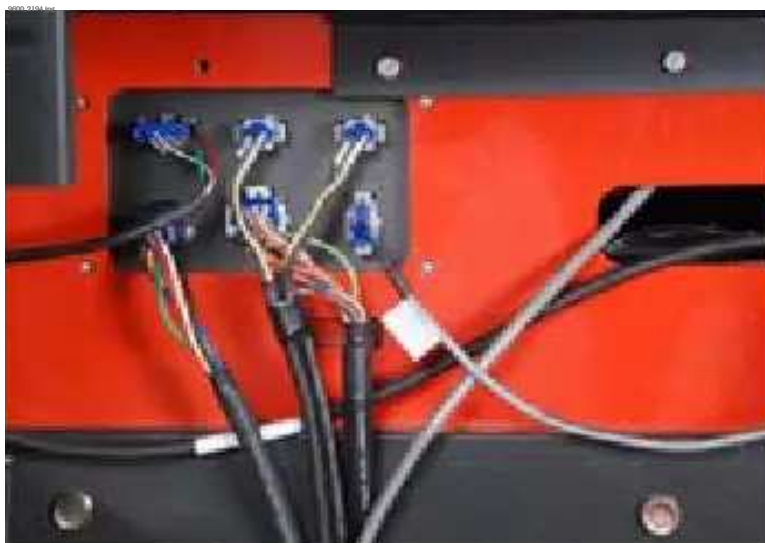
Figure 3-9. Mast to Tractor Cable Connections
