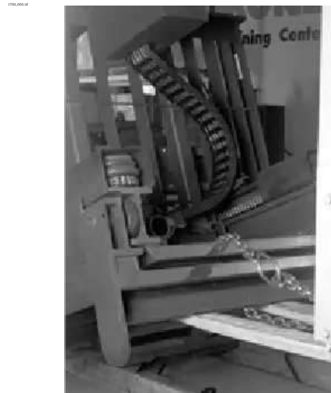
Figure 3-3. 9600 Mast Erection Using Lift Truck
