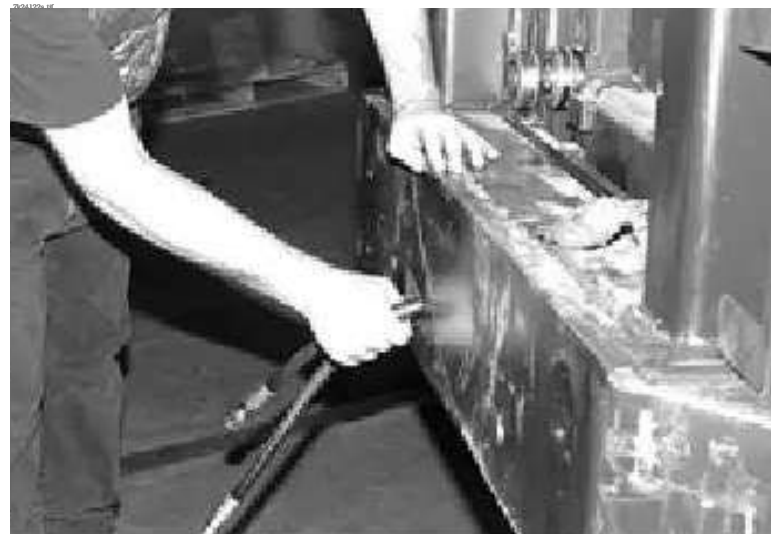
Figure 3-7. Pulling Hydraulic Hoses Through Mast
