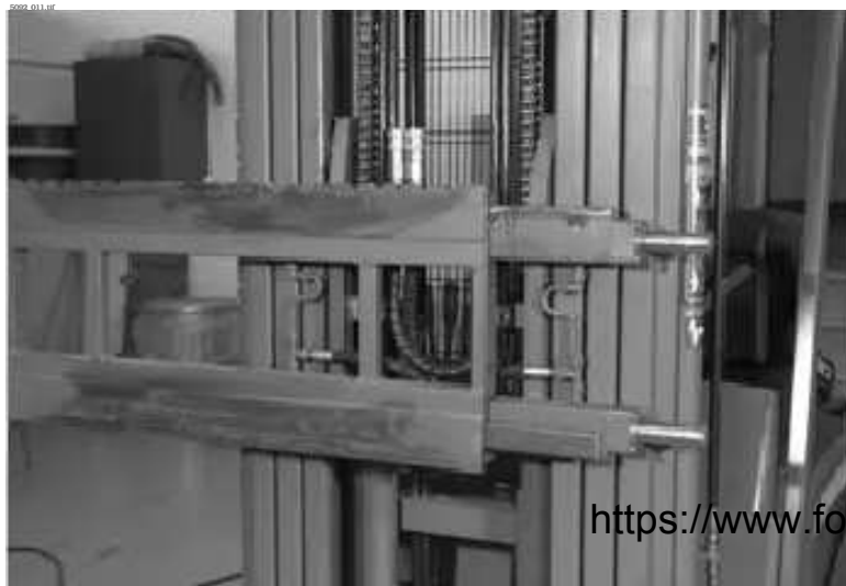
Figure 7-62. Carriage Frame Partially Removed
