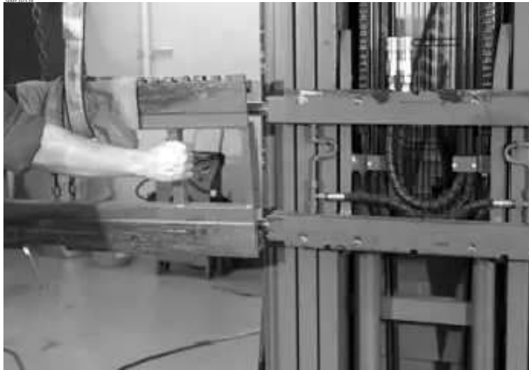
Figure 7-65. Carriage Frame Installation
