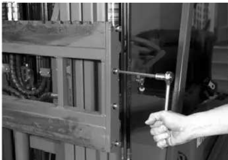
Figure 7-61. Example of Side Plate Bolt Removal
