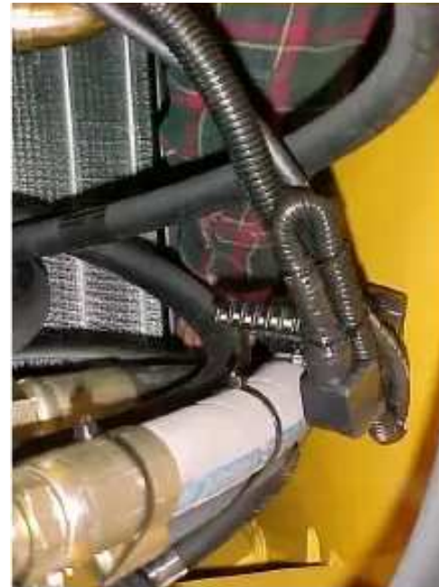
INSTALLING LEFT RADIATOR MOUNT
