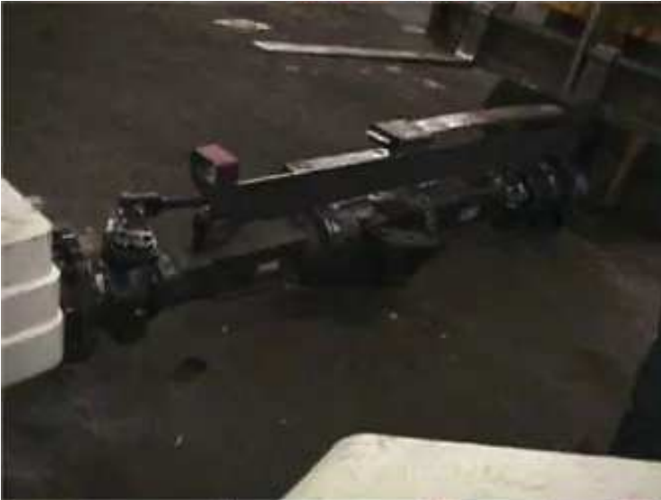
MOVING REAR AXLE INTO PLACE
