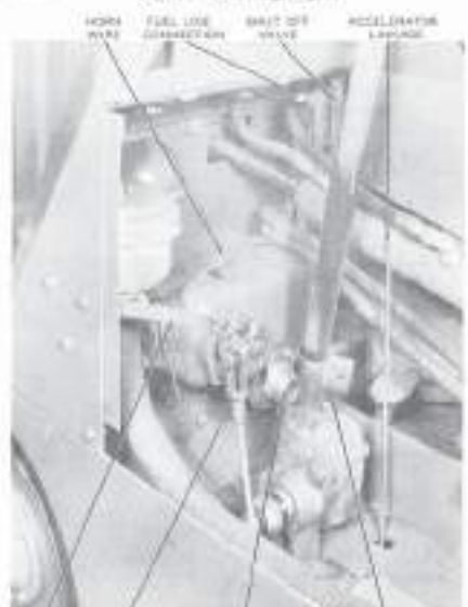
Fig. 8. Front Department of Chassis with Engine Mounted
